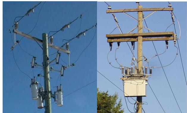
Fig. 2. Single-phase (left) and three-phase (right) pole-mounted reclosers.
